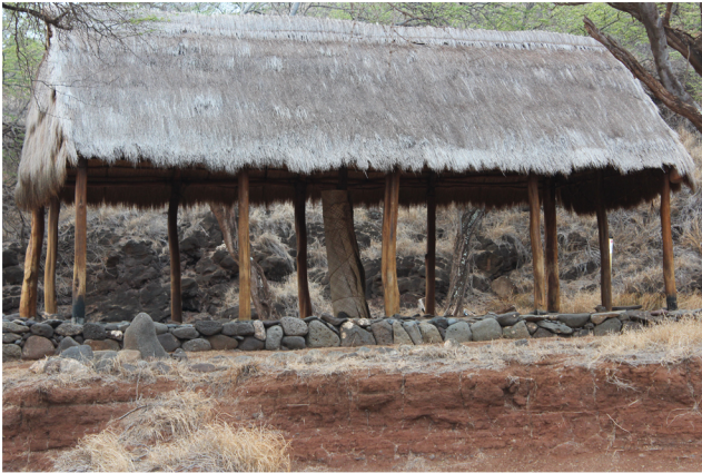
Namakapili, the name for the hale hālāwai or meeting house, in Hakioawa was completed in 2009. This hale is a testament of the 'Ohana's dedication to their relationships with the general community and Kaho'olawe.
